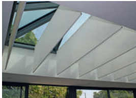
Ceiling and baffles - Restaurant (FR)
